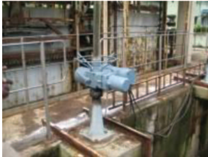
Figure 3.7 Electric motor driven gear actuator
