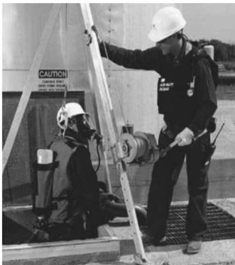
Figure 9.8 Photo showing typical confined space entry
