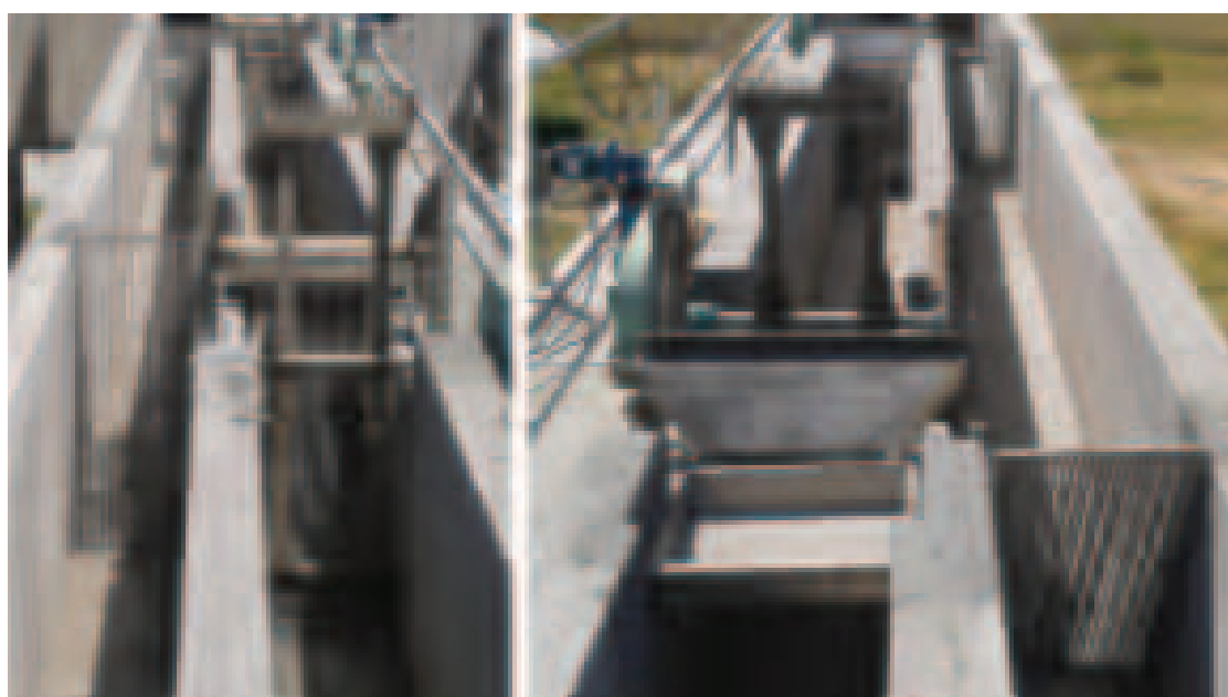
Figure 3.12 UNIDO type arc screen
